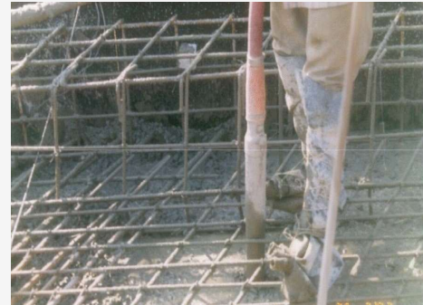
Compaction by vibrator
