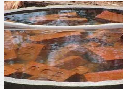
Soaking of bricks
