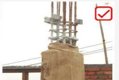
Proper use of Cover block
