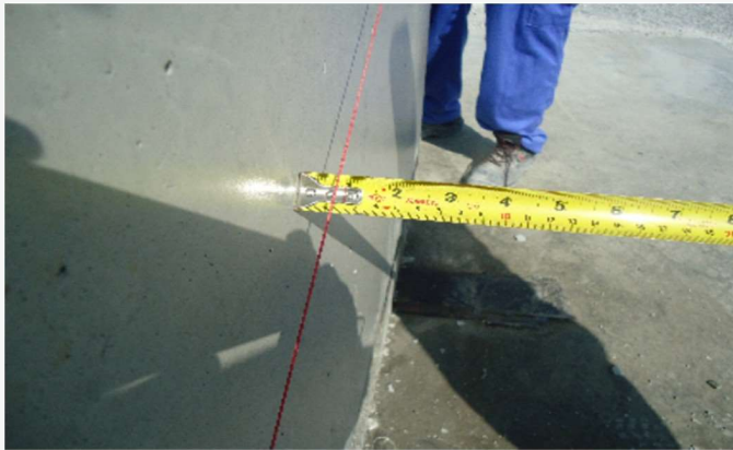
Formwork Deviations
