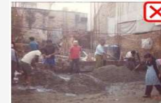
Concrete mixing manually with poor quality
