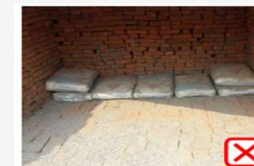
Cement stored in ground above brick soling
