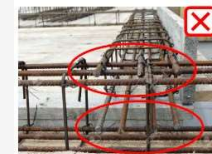
Insufficient Development Length
