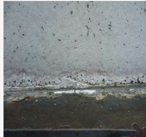
Slurry leakage
