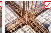
Reinforcement of beam confined by column reinforced
