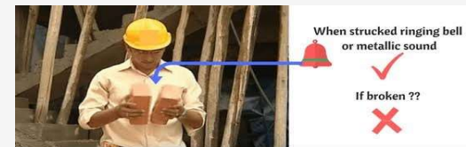
Checking quality of brick on site
