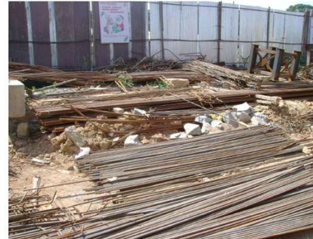
REINFORCEMENT YARD IN BAD SHAPE
