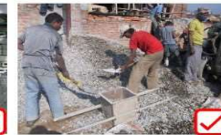
Measurement of Ingredients by standard box
