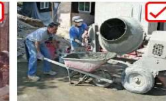
Concrete mixing by machine
