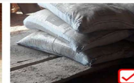
Cement stored above wooden plank
