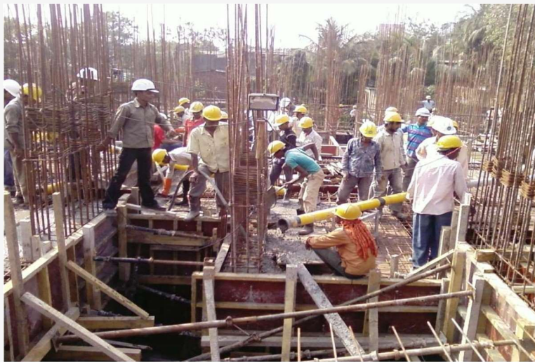
Slab & Beam Formwork
