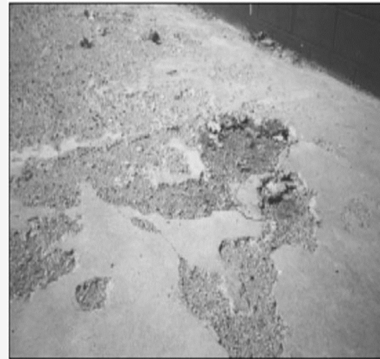
Poor surface finish
